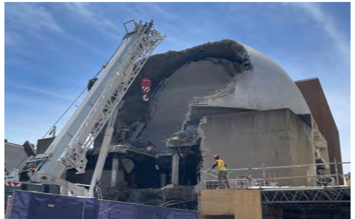
Demolition of the former McLaughlin Planetarium, May 12, 2026
